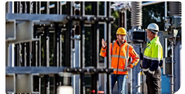
Maasbracht high-voltage substation extension
